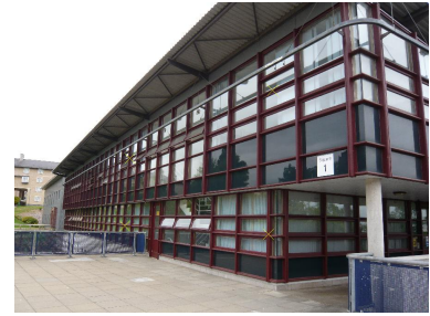
(a) A photograph showing the normal foreshortening due to distance, with four points marked on features that lie on the side of the building
